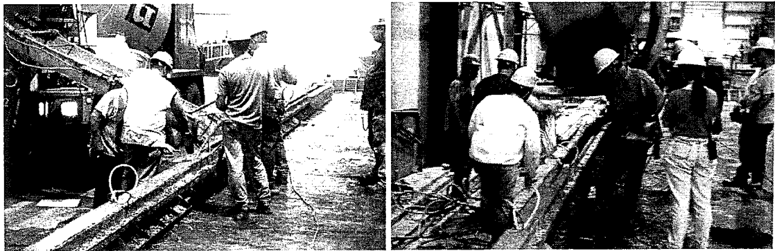
Figure 7-6: Placement of Web Concrete
