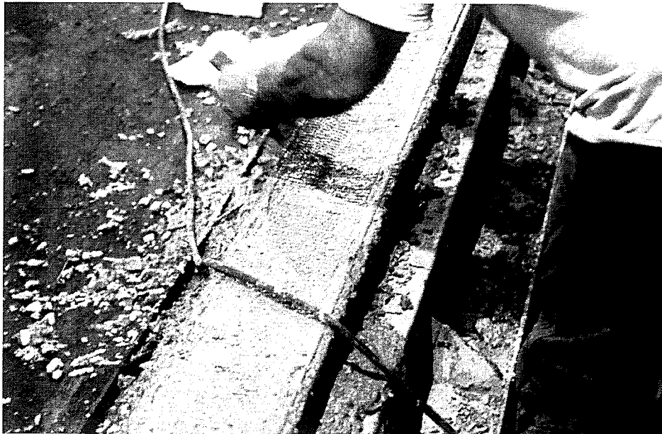
Figure 7-12: Applying the Rake Surface Finish
