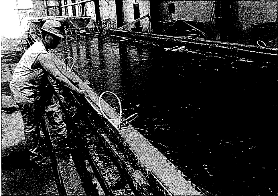
Figure 7-10: Applying the Broom Surface Finish
