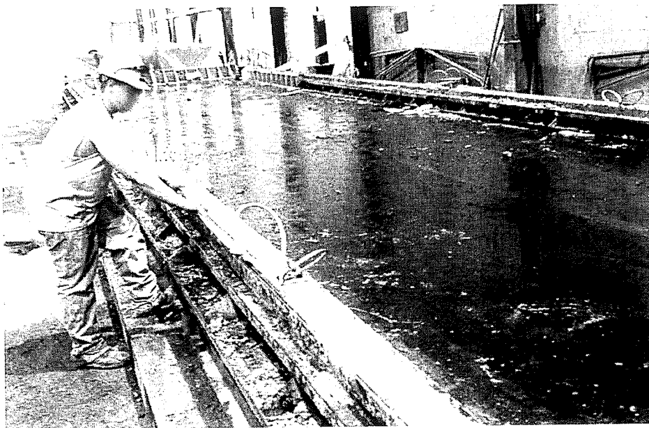
Figure 7-10: Applying the Broom Surface Finish
