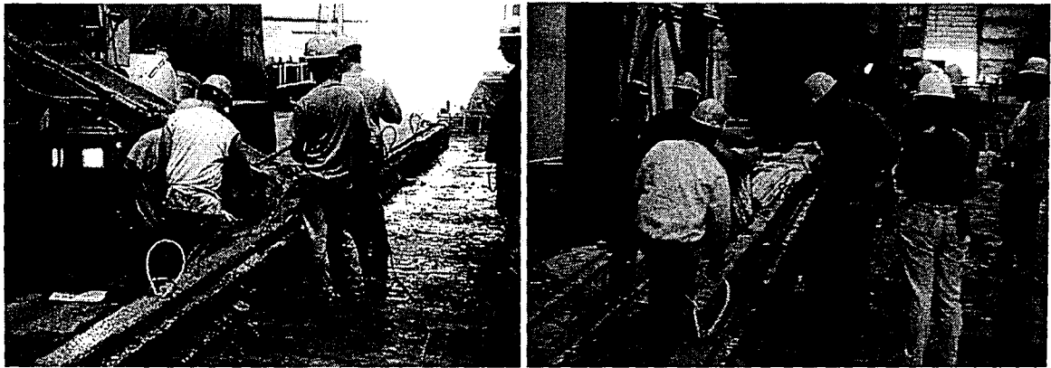
Figure 7-6: Placement of Web Concrete
